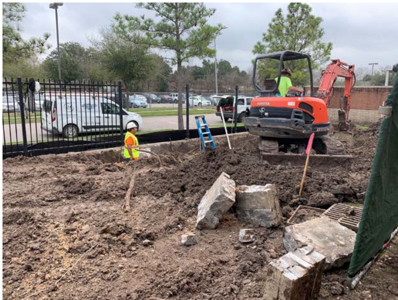
Playground equipment removed for installation of new storm lines
