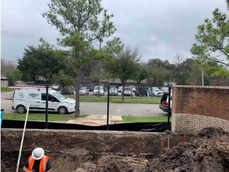
Trenching for new storm lines at playground area.
