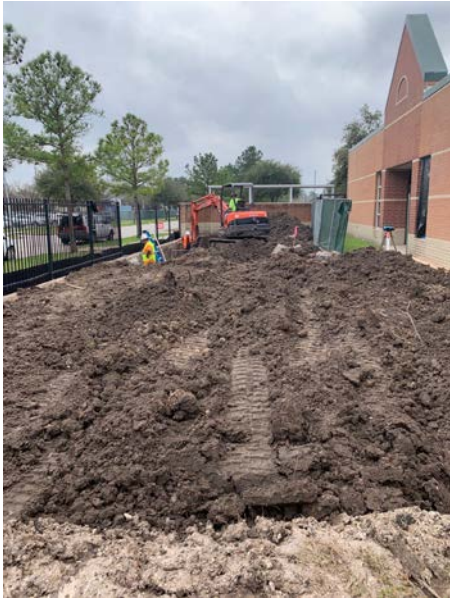
Installing new storm lines at playground area
