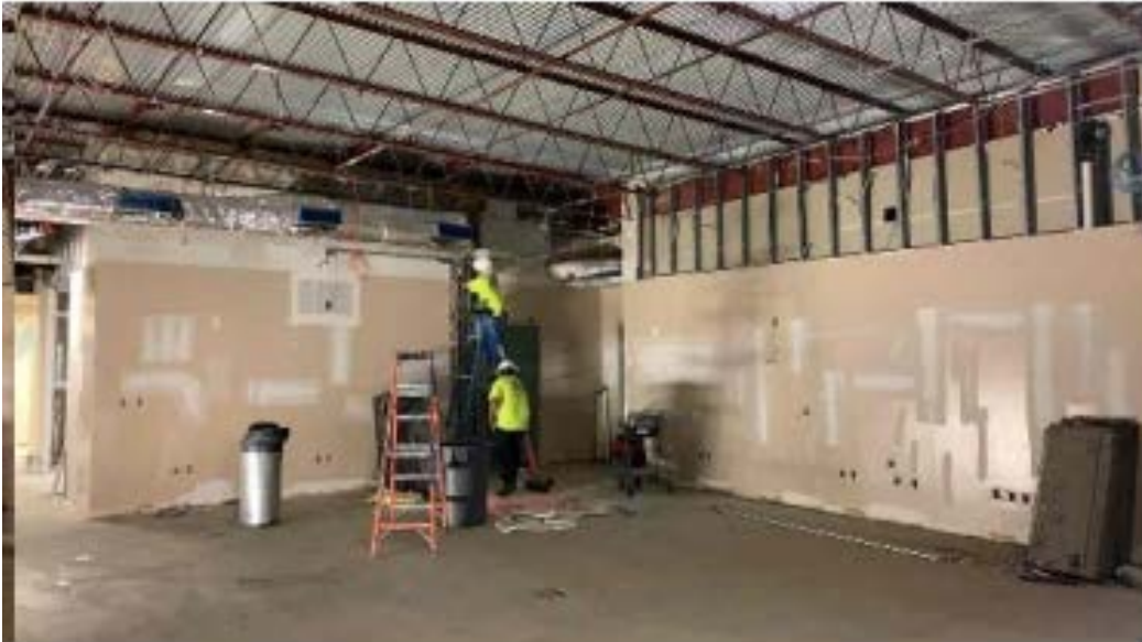
Re-routing MEP at Collaboration Spaces
