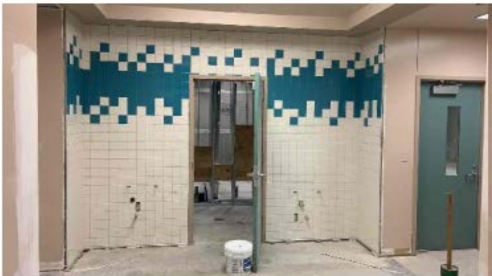
Install new tile at drinking fountains
