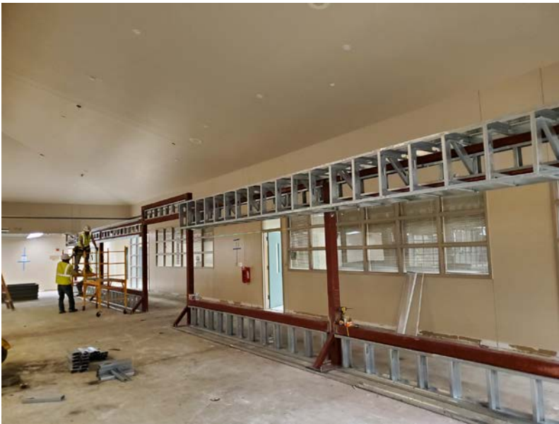
Framing window wall and benches at Library
