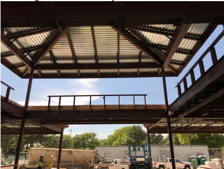
Installing Structural Framing for Pop ups
