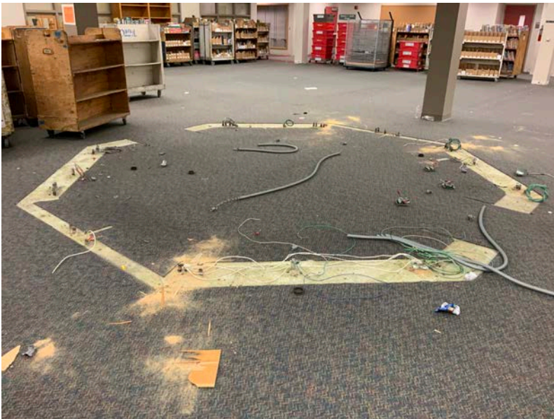
Removing casework in Library
