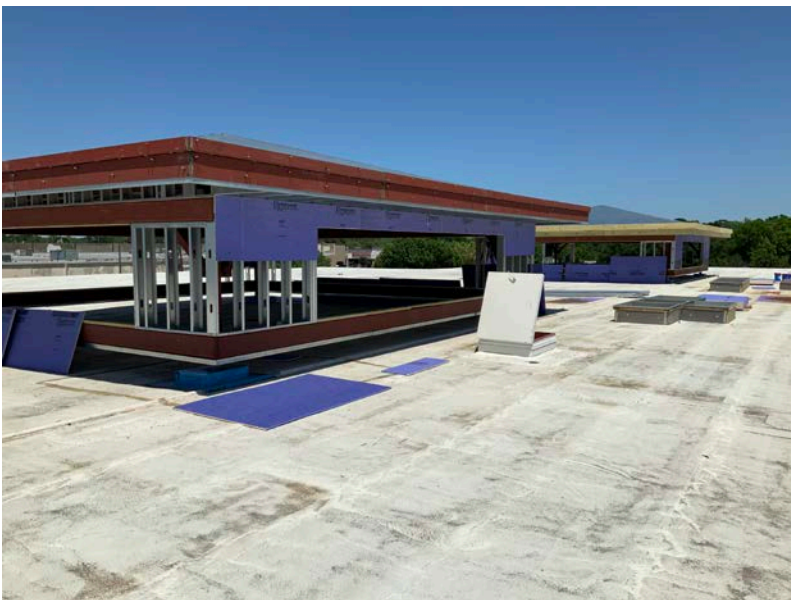
Completing framing and close in at structural pop-ups
