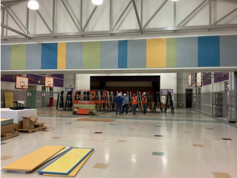
Installation of acoustical panels completed
