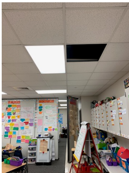
Removing ceiling tiles for above ceiling work
