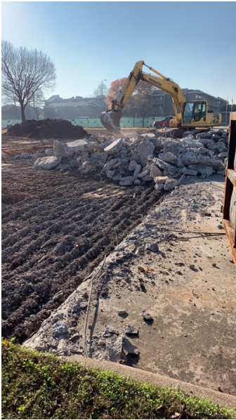
Existing parking lot being removed
