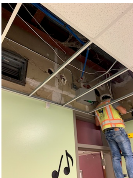
Above ceiling mechanical work starting
