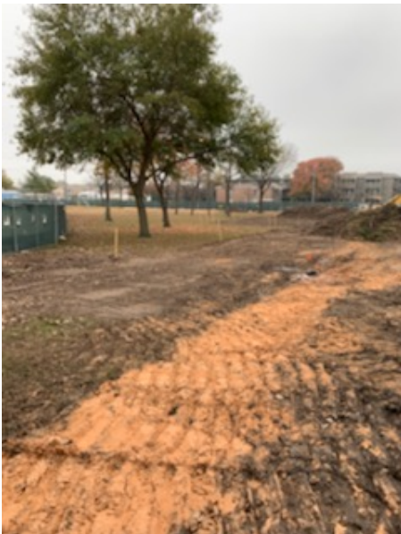
Clearing site for construction of New Addition
