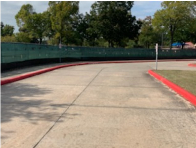
Construction and silt fencing installed at exit of parent drop off
