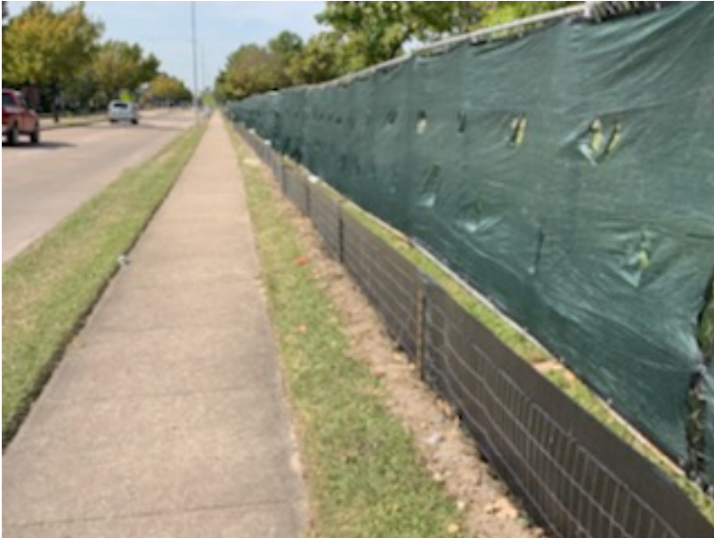
Construction and silt fencing installed along Hammerly
