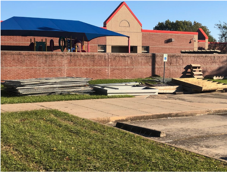
Construction fencing materials laydown area
