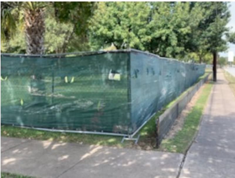
Construction fencing installed along Ojeman
