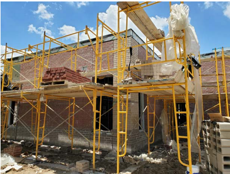
Completing masonry at new addition
