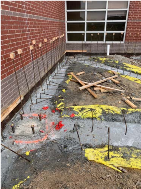
Exterior Grade Beams Poured at New Addition
