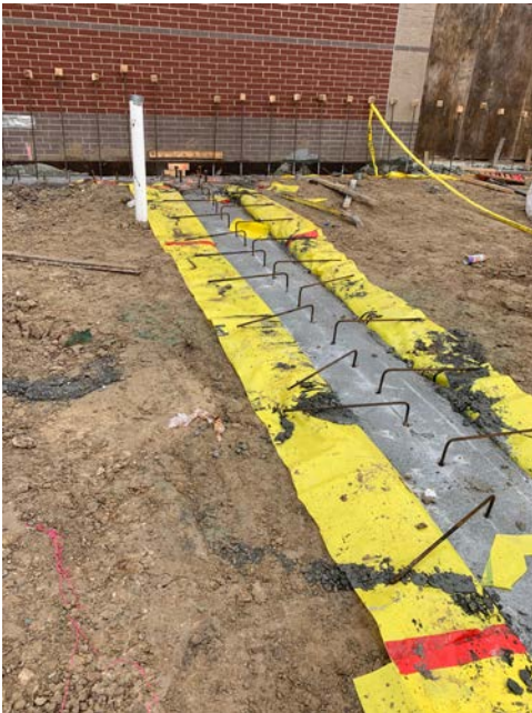
Exterior Grade Beams Poured at New Addition
