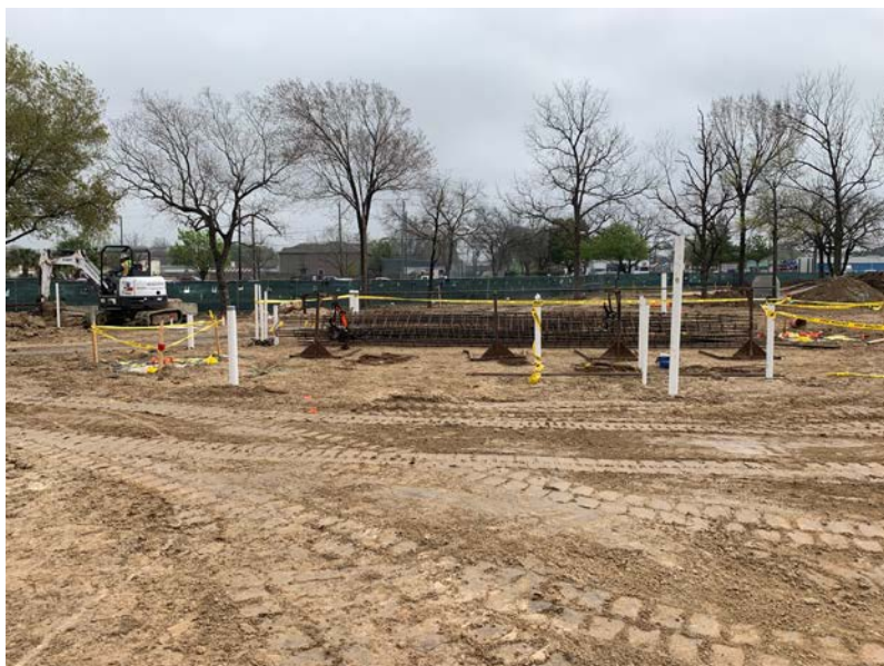
Drilled Piers and Plumbing Stub-ups Completed
