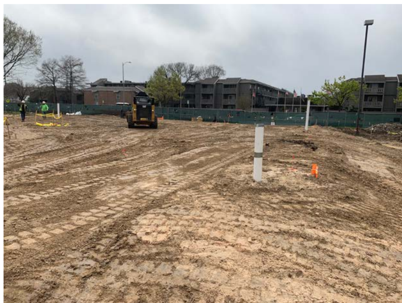
Drilled Piers and Plumbing Stub-ups Completed
