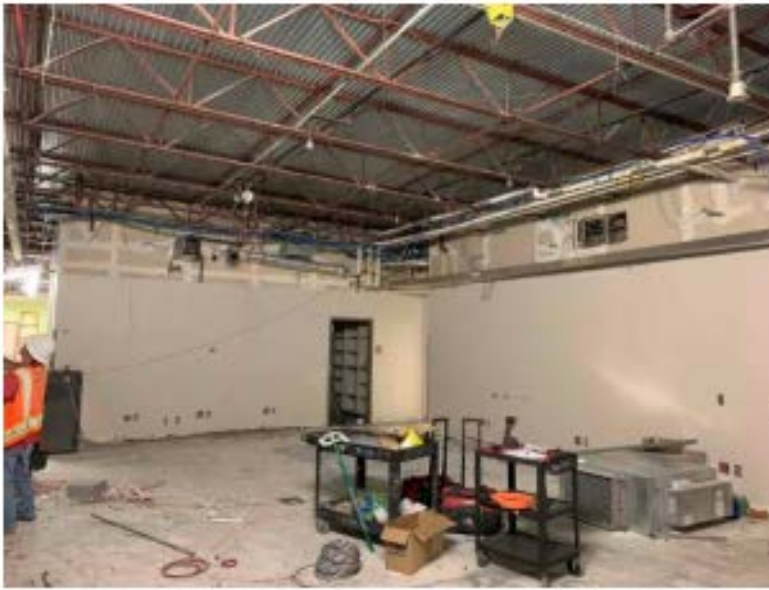
Re-routing existing MEPT at Collaboration spaces
