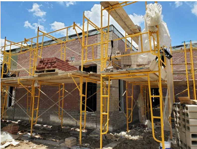
Completing masonry at new addition
