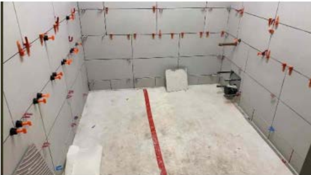
Installing new tile at restrooms
