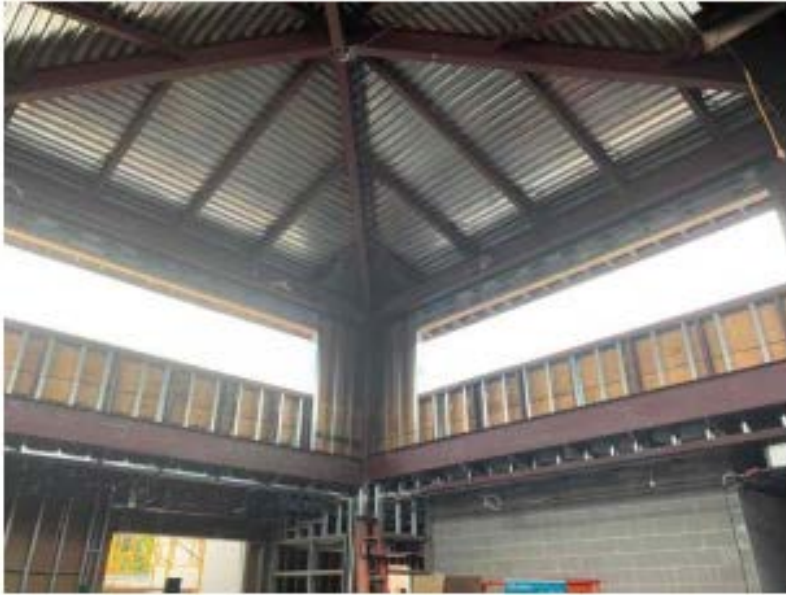
Framing new windows at new addition structural pop-up
