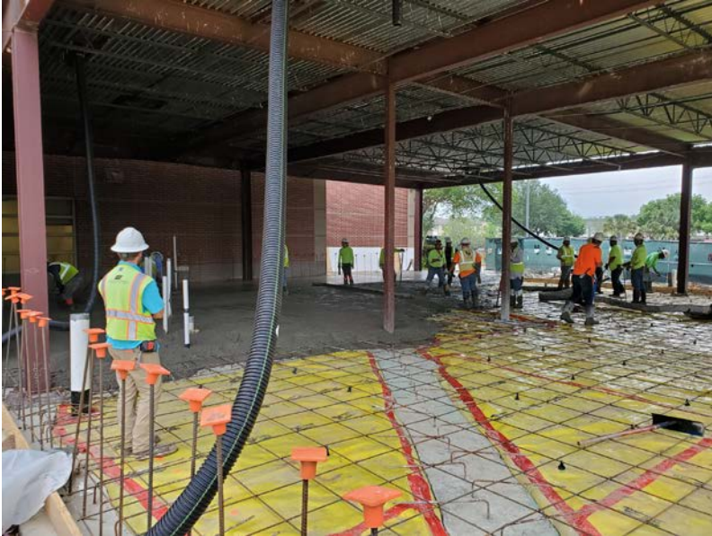
Pouring slab at New Addition
