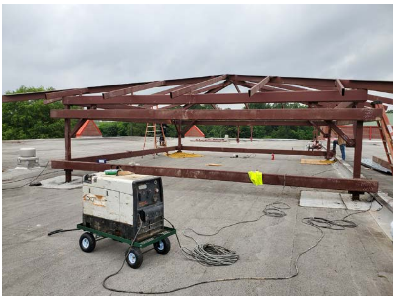
Completing welding at structural pop-ups Area 2
