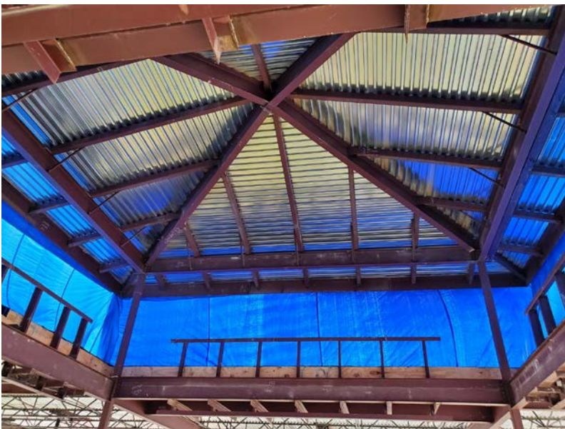
Metal decking complete at structural pop-up
