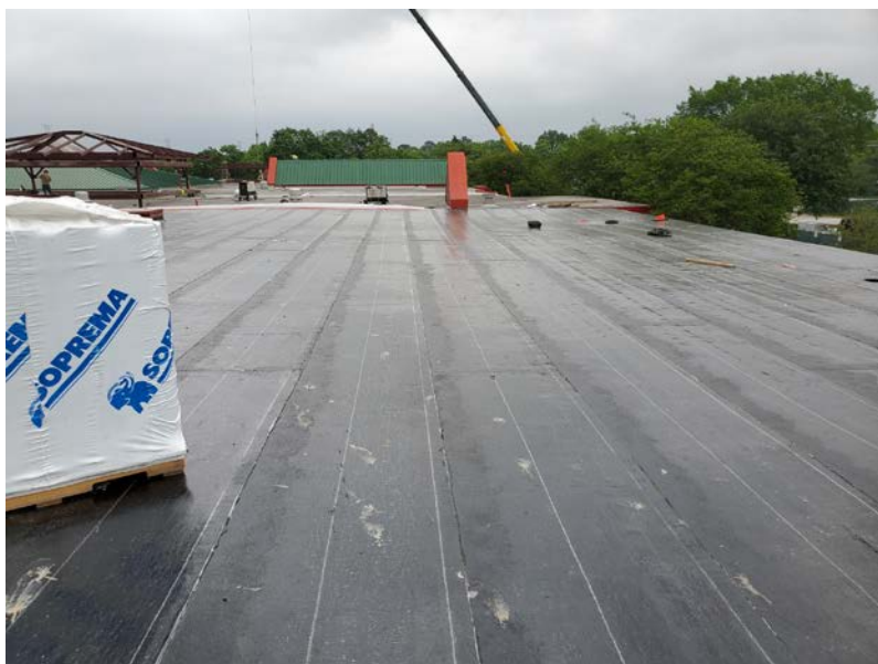
Roofing base sheet installed at New Addition
