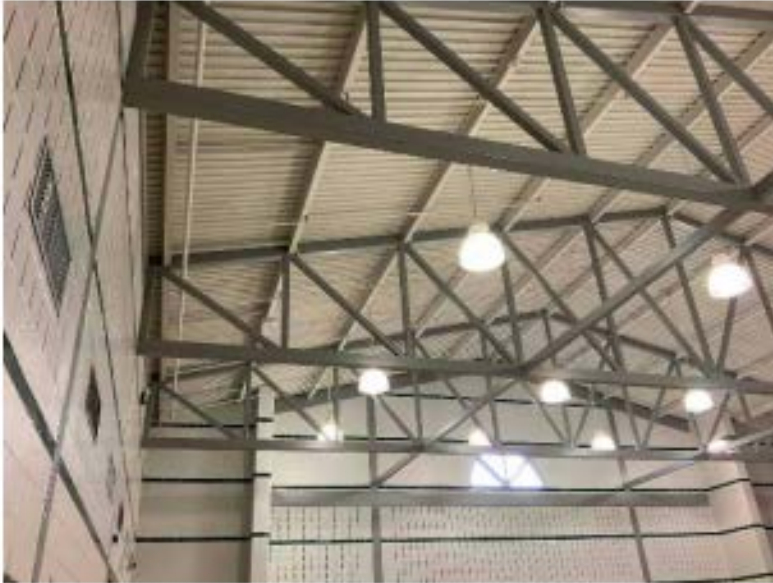
Interior painting in Gym and Cafeteria started
