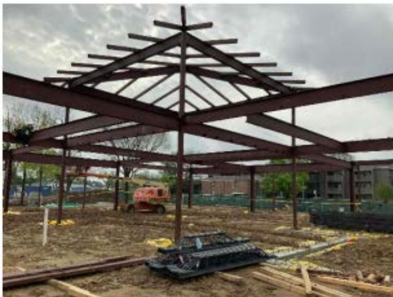
Structural steel started at New Addition
