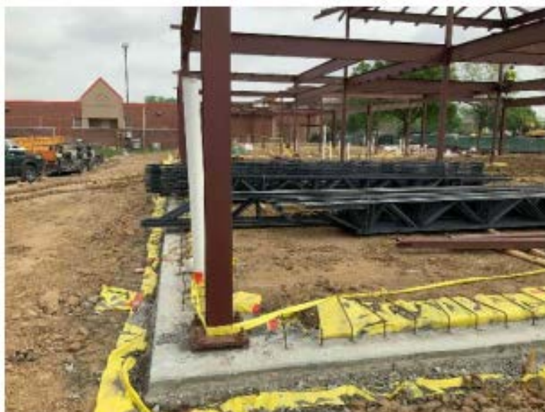
Structural steel started at New Addition
