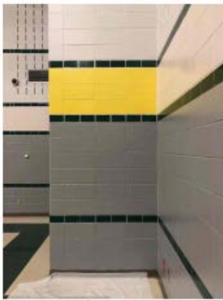
Interior painting in Gym and Cafeteria started
