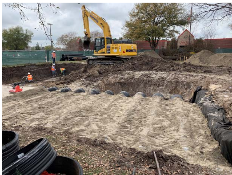
Installation of piping for detention under new teachers parking
