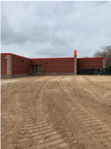
Site cleared for New Addition
