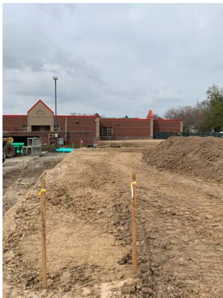
Building pad for New Addition placed
