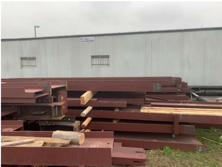
Structural steel delivered to site for New Addition
