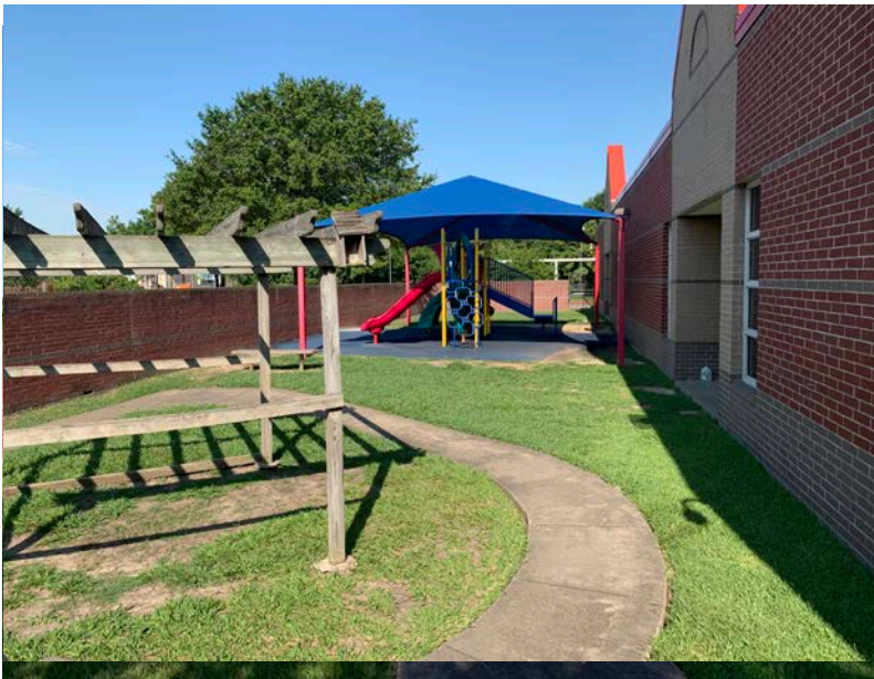
CM@R Confirming Existing Conditions at Playground
