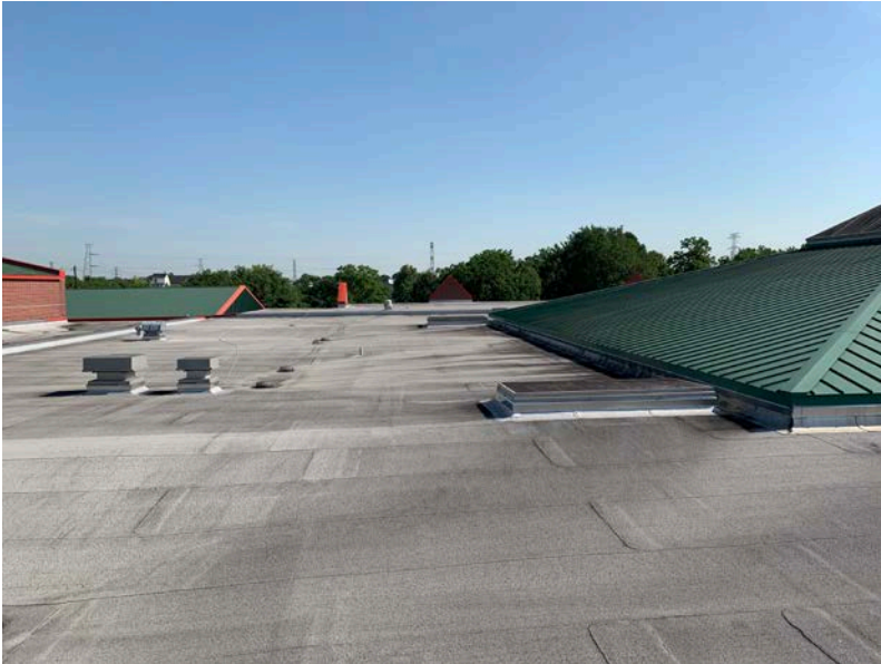
Roofing Site Walk with CM@R.
