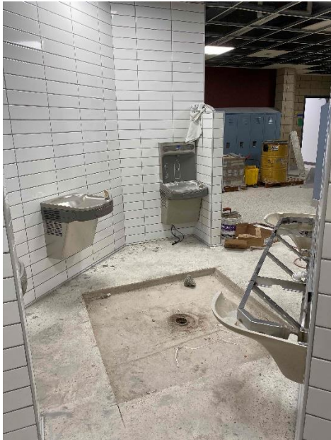
CCES – Fixtures mounted in area A washroom
