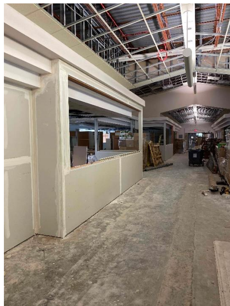
CCES – Drywall nearly complete for secure media center
