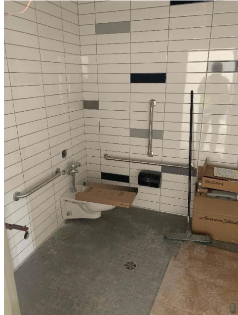
ECFC – New private bathroom in area A nearly complete
