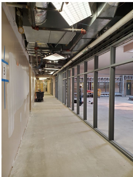
Installing new window wall at Library
