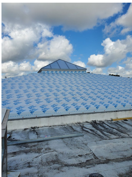
Installing standing seam roof panels at Library roof
