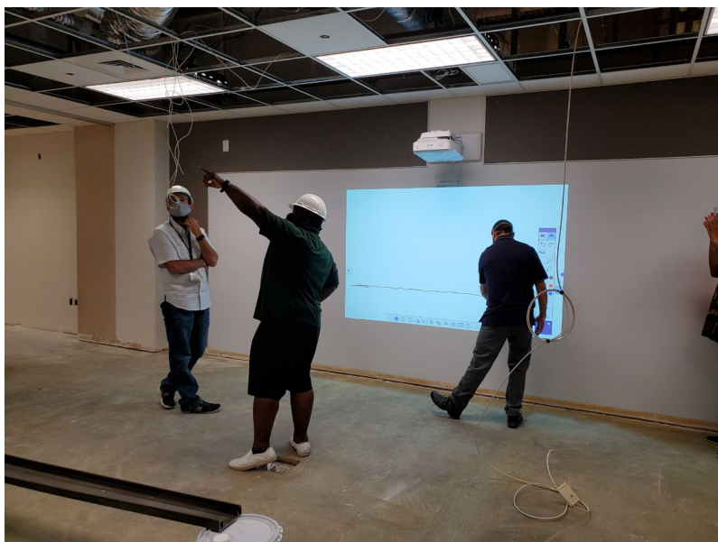
Installing new teaching walls at classrooms
