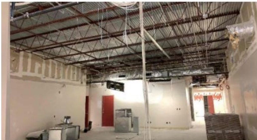
Re-routing MEP at Collaboration Spaces
