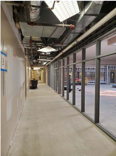
Installing new window wall at Library
