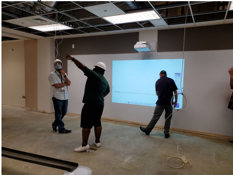
Re-routing MEP at Collaboration Spaces
