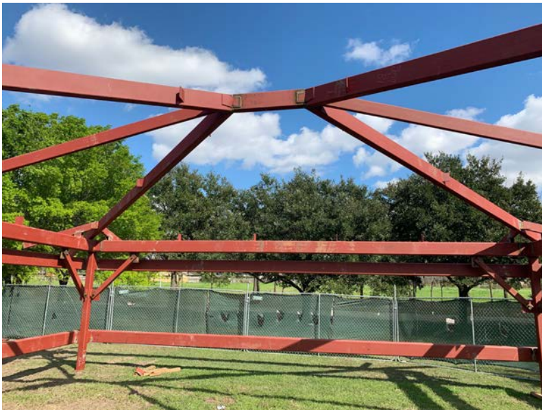
Completing Fabrication of Structural Steel for Pop-ups
