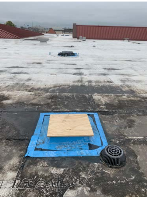
Installed Curbs for Pop-pups
