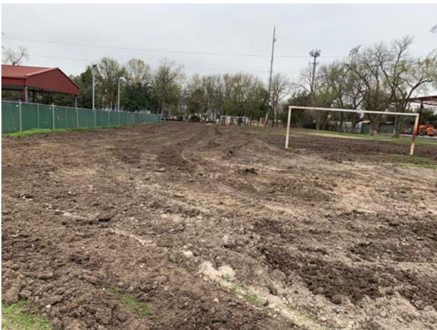
Grading at Soccer Field 2017 SBISD Bond Facility Name: Buffalo Creek Elementary
