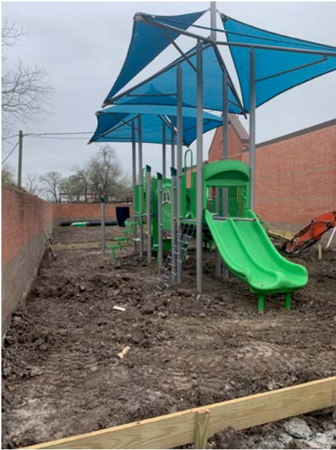
Preparing Grading for Fall Protection
