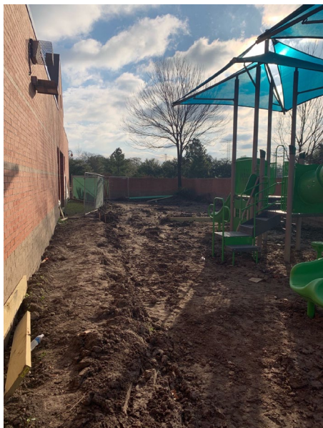
Installation of new storm lines at playgrounds
