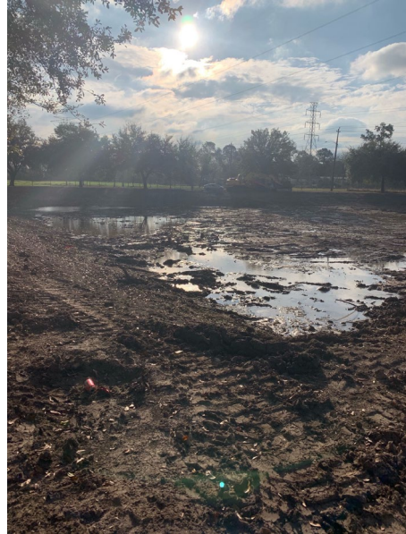
Re-grading at existing detention pond
