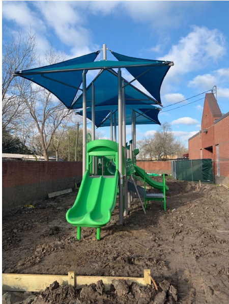
New playground equipment installed
