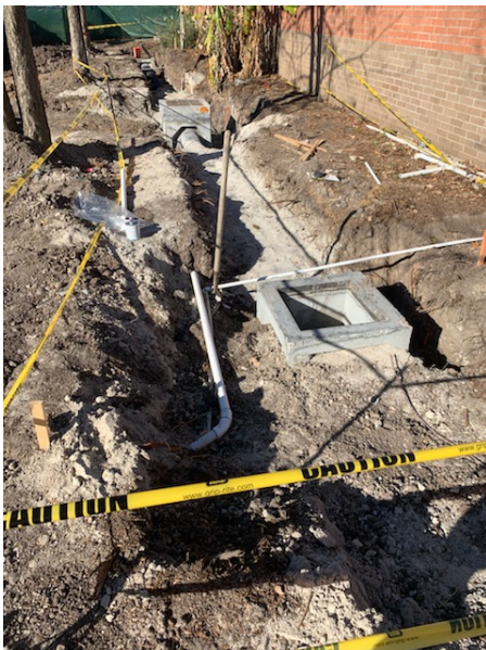
Backfilling at new storm line
