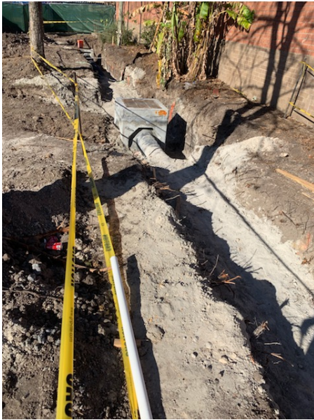
New storm inlet in place
