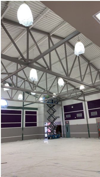
Painting interior of cafeteria
