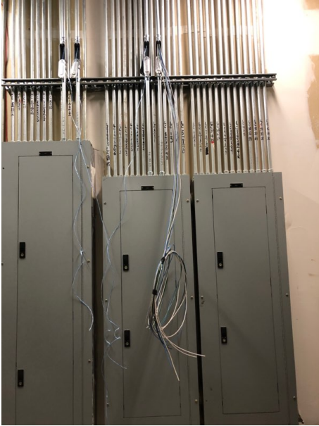
New circuits being pulled to electrical panels
