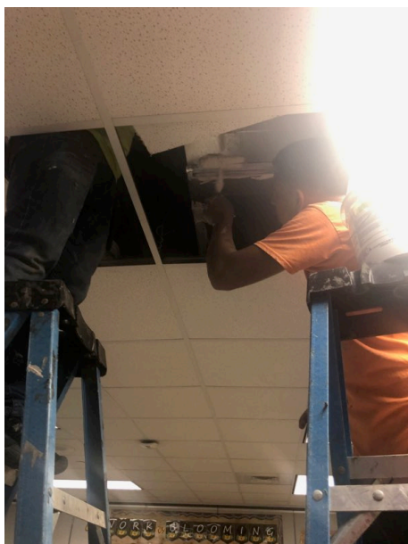
Above ceiling mechanical work
