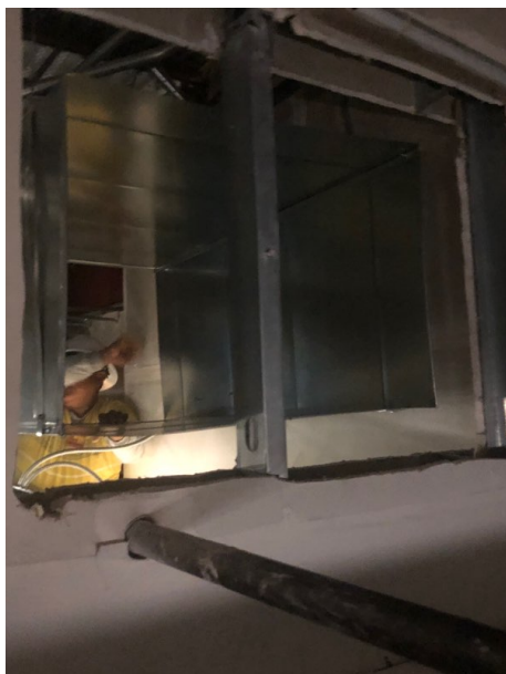
After-hour mechanical work started
