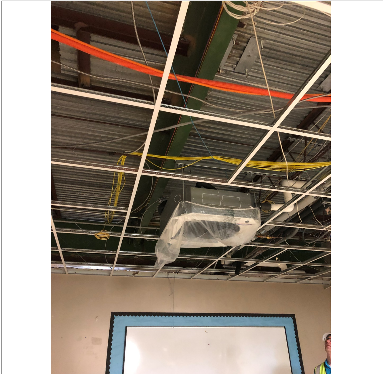
New HVAC units in place.
