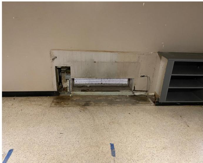
Old pipe removal during Phase 5. Wall will be patched and floor will be clean and patched.
