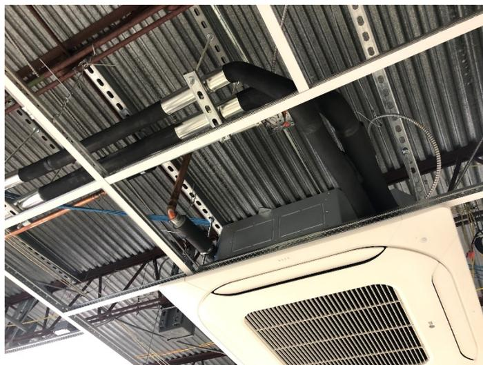
A look of the new HVAC “in classroom” unit and it’s piping. It is smaller and much less noisy that the original system.
