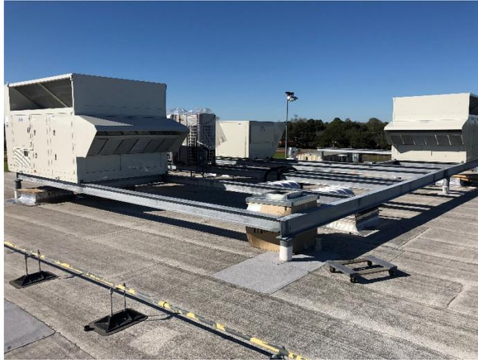
Install of new rooftop units for Phases 3 and 4. The steel the units are sitting on where added to the structure as a part of this project.
