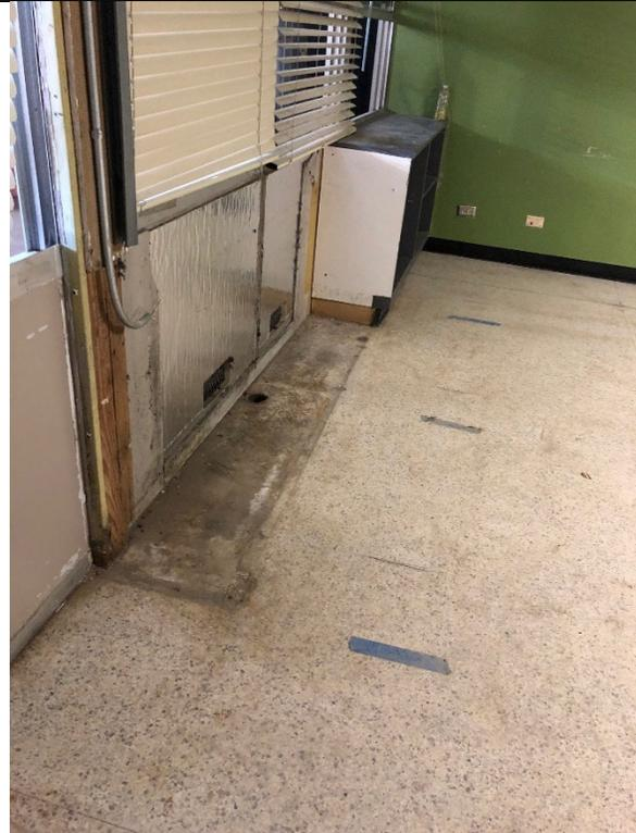
Old unit vent in classroom has been removed. The area will be cleaned, and new infill material will be installed in its place for a clean and nice look.
