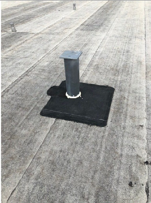
Steel on roof for new mechanical units
