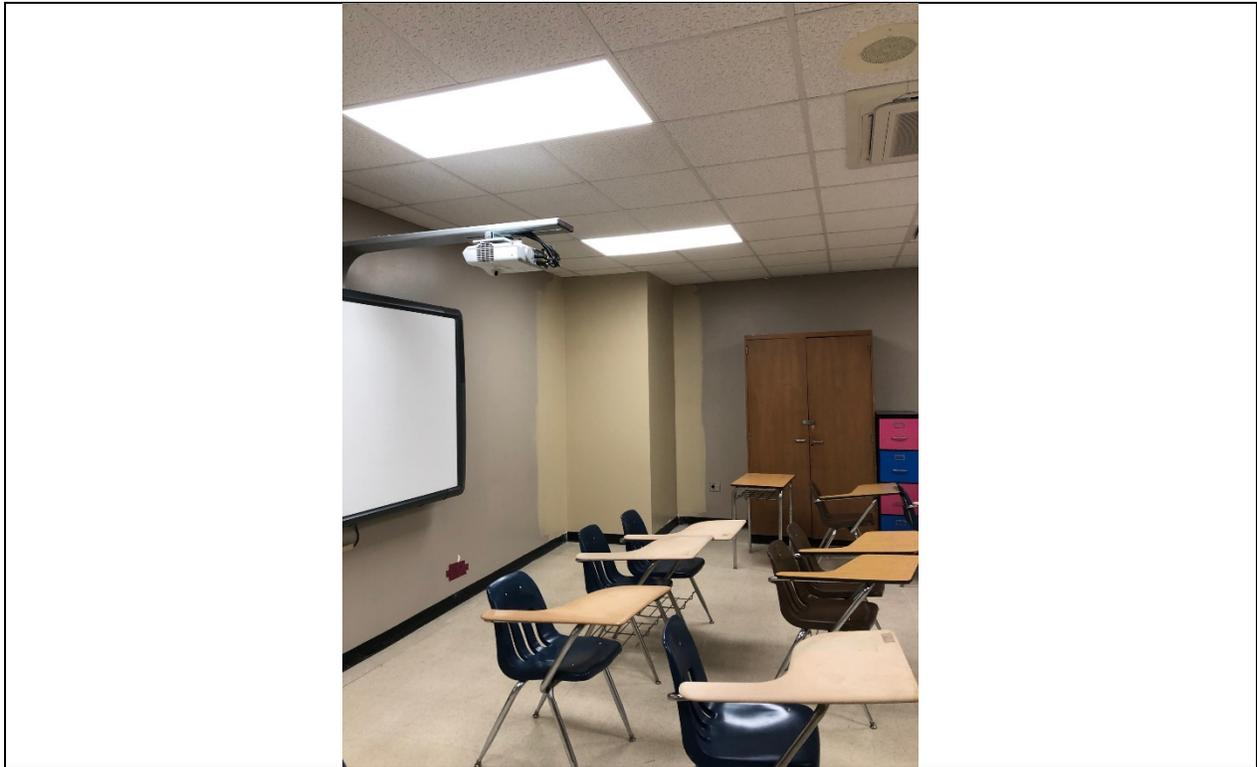
Picture shows a new chase in a classroom. This chase will allow for cool air for the first floor classrooms. The paint will match the existing walls.
