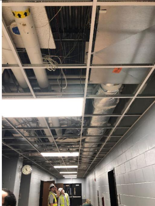
Area H Locker Room Corridor ducting has been installed, and ceilings will be installed shortly.
