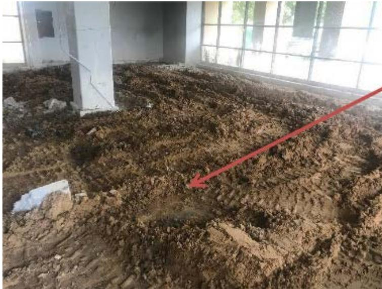
Slab has been removed, graded, and prepared for the new floor.
