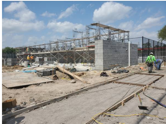
Tennis Field House CMU Walls
