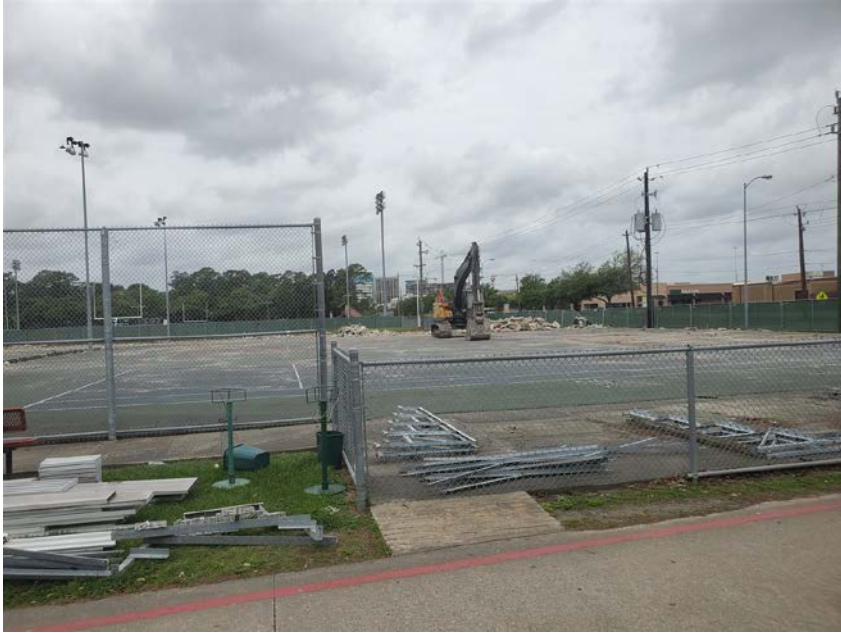
Removal of Old Tennis Courts
