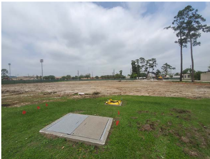
Prepping site for new building
