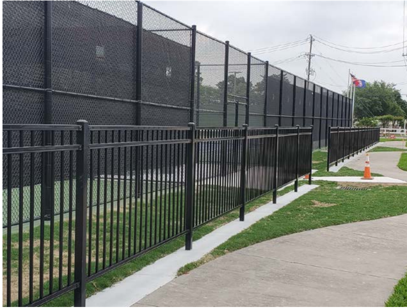
Ornamental fencing at new tennis courts
