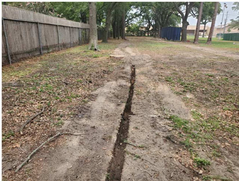
Root Pruning at existing trees for protection
