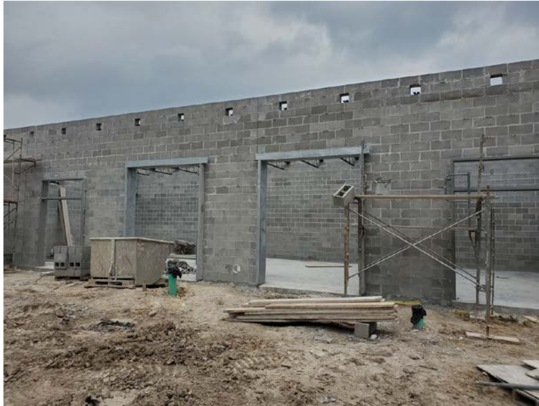
Exterior wall at new tennis field house
