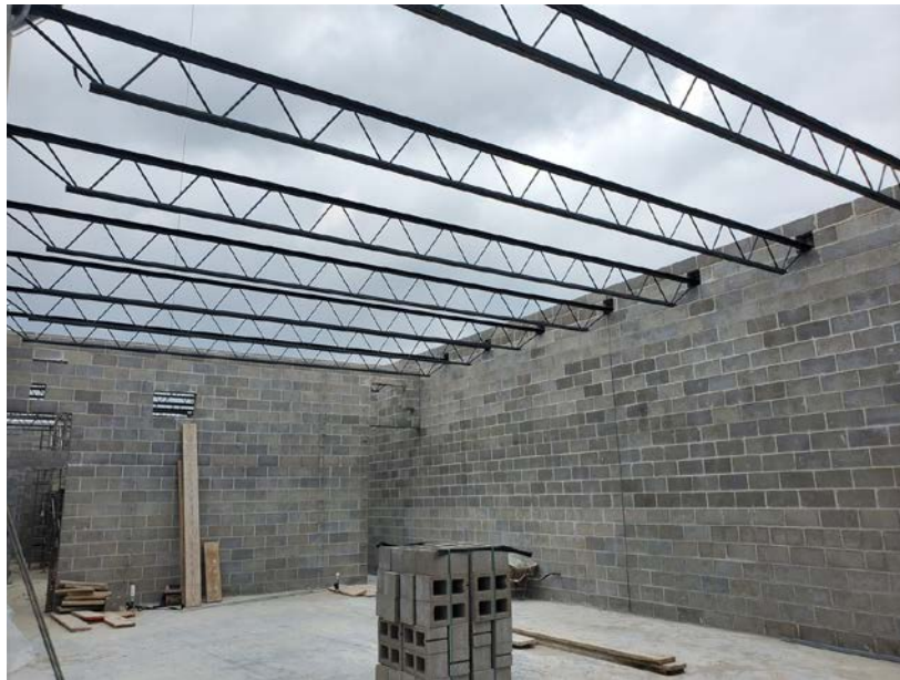
Steel erection at new tennis field house
