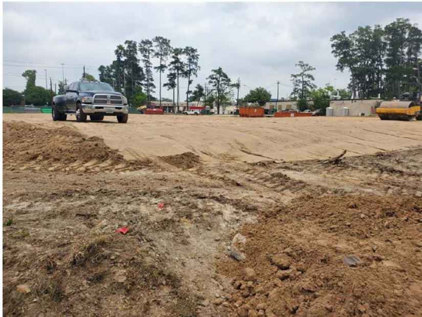
Building Pad for new building
