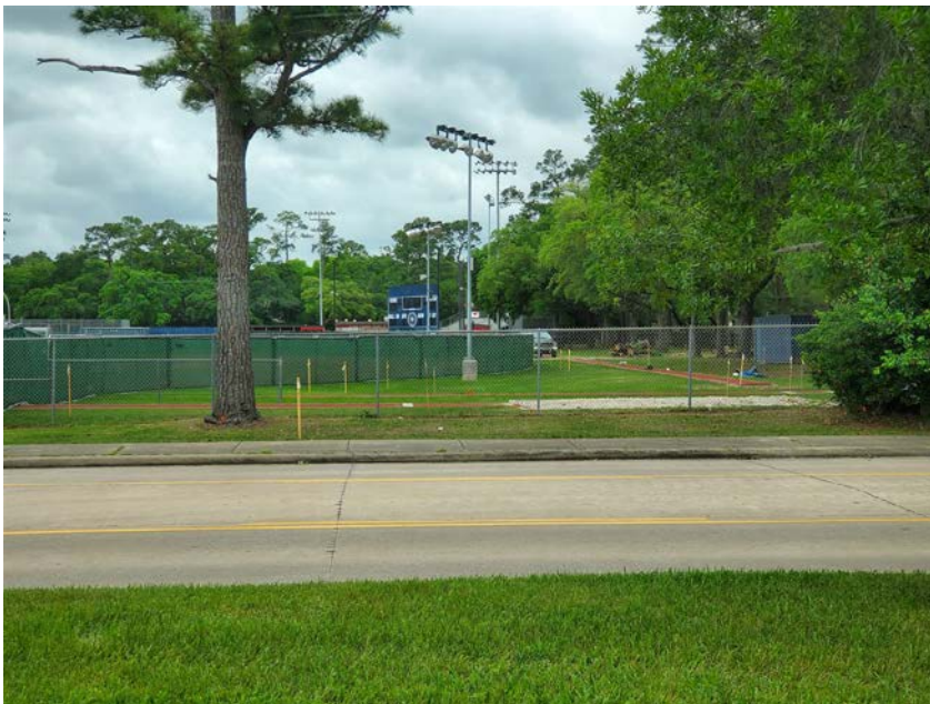
Prepping for new driveway and storm line
