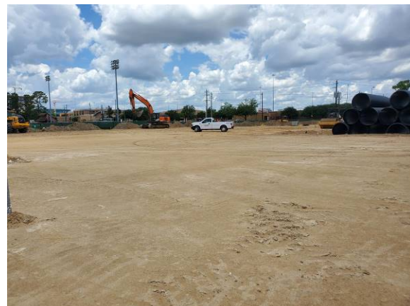
New Building Pad
