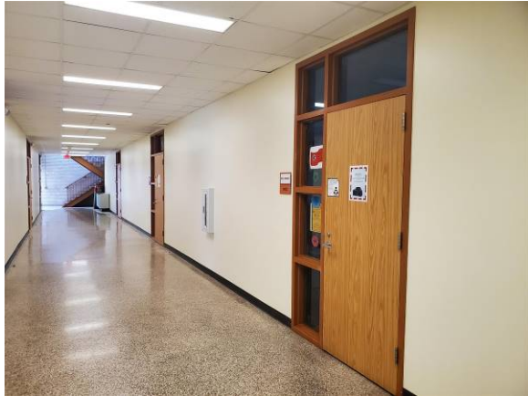
Existing walls and frames repainted
