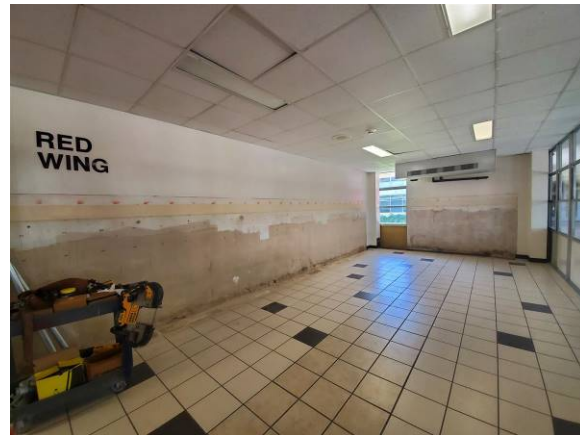
Existing locker removal and painting
