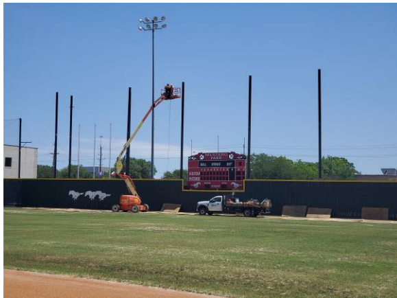
Installing net poles at Baseball
