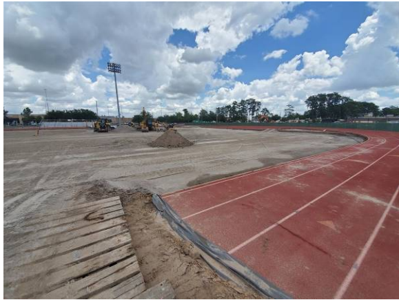
Turf field old grass and base removed
