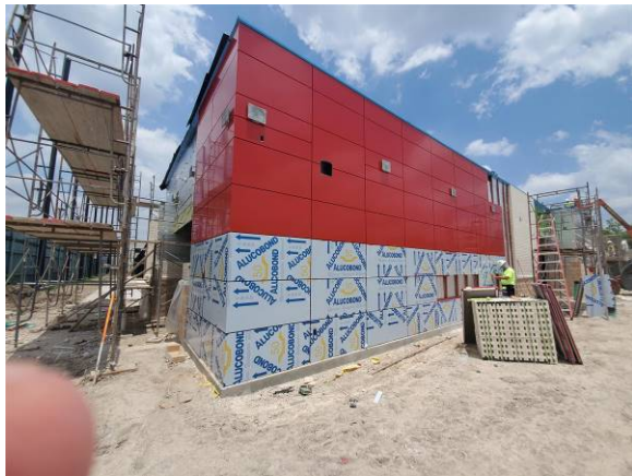
Tennis building metal panel
