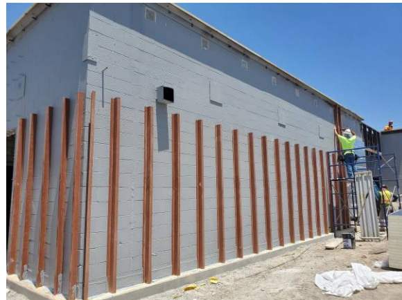
Installing metal panels at Tennis building
