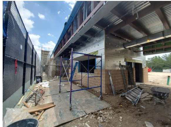
Tennis Building Coach's Office
