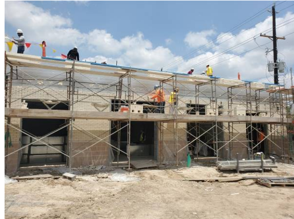
Tennis Building masonry and roofing
