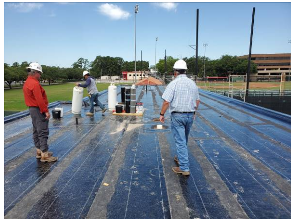
Tennis building roof water testing
