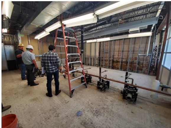
Existing Toilet Renovations
