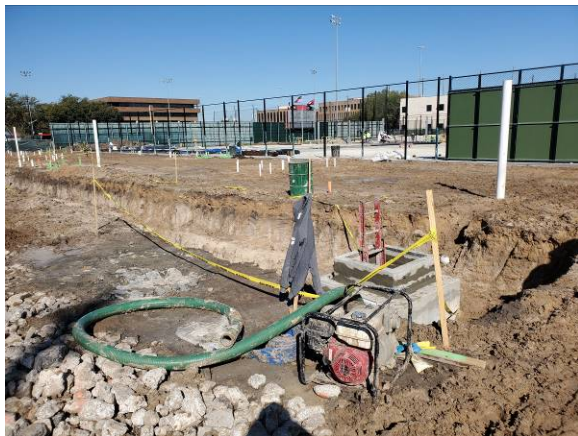
Storm Drainage south of the Tennis Building
