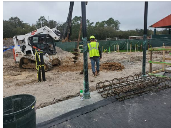
Drilling Piers for the Tennis Building
