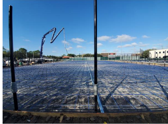
Tennis Court Slab Prep
