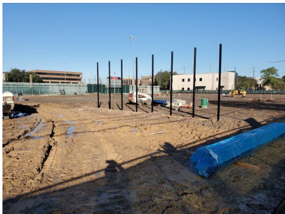
Setting tennis court poles
