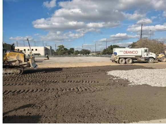
Subsurface prep for Tennis Field House
