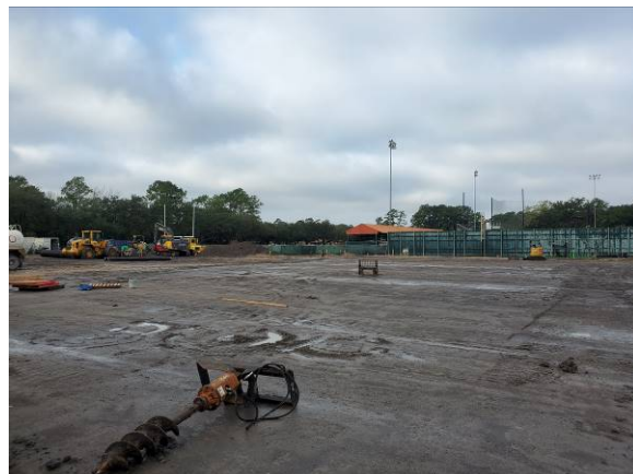
Subsurface prep for Tennis Courts
