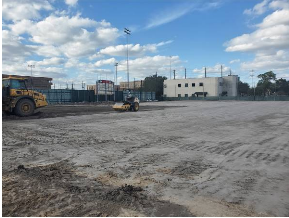
Subsurface prep for Tennis Courts
