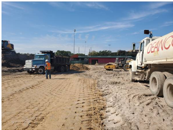
Building pad foundation for Tennis Field House
