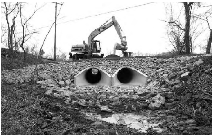
Abbott Road Culvert Replacement
