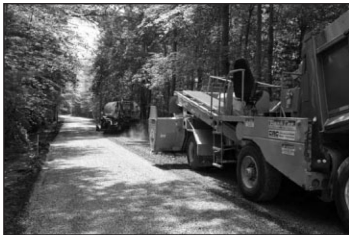
Chip seal operation on Wheelock Road
