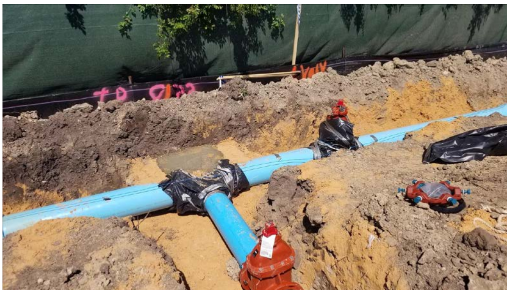
Underground utility piping installation
