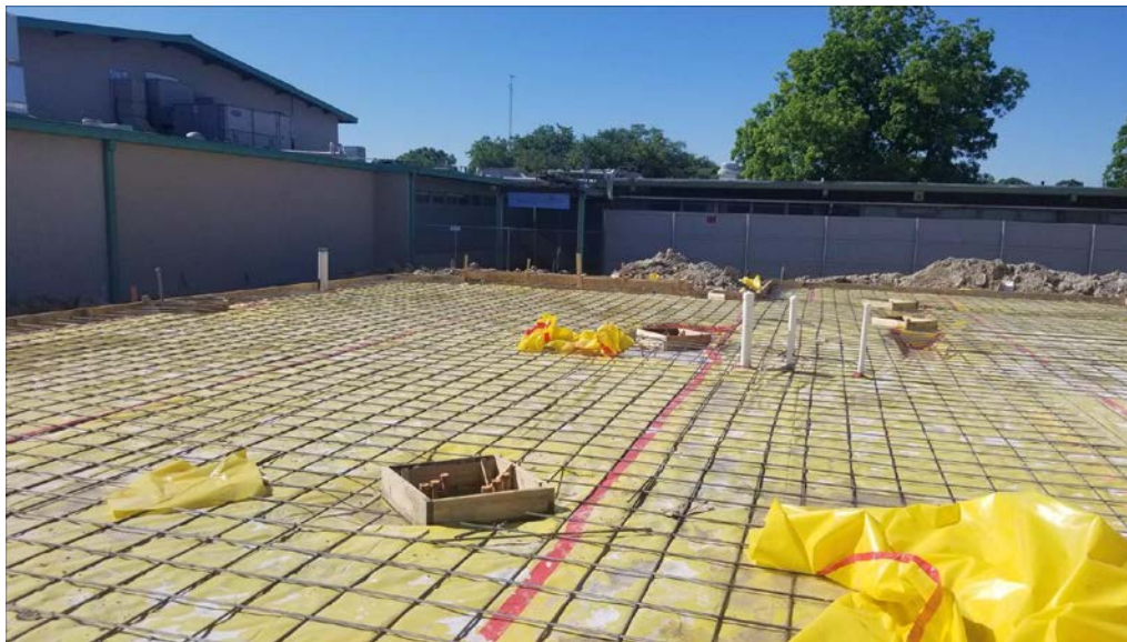
Slab preparation work in Area A
