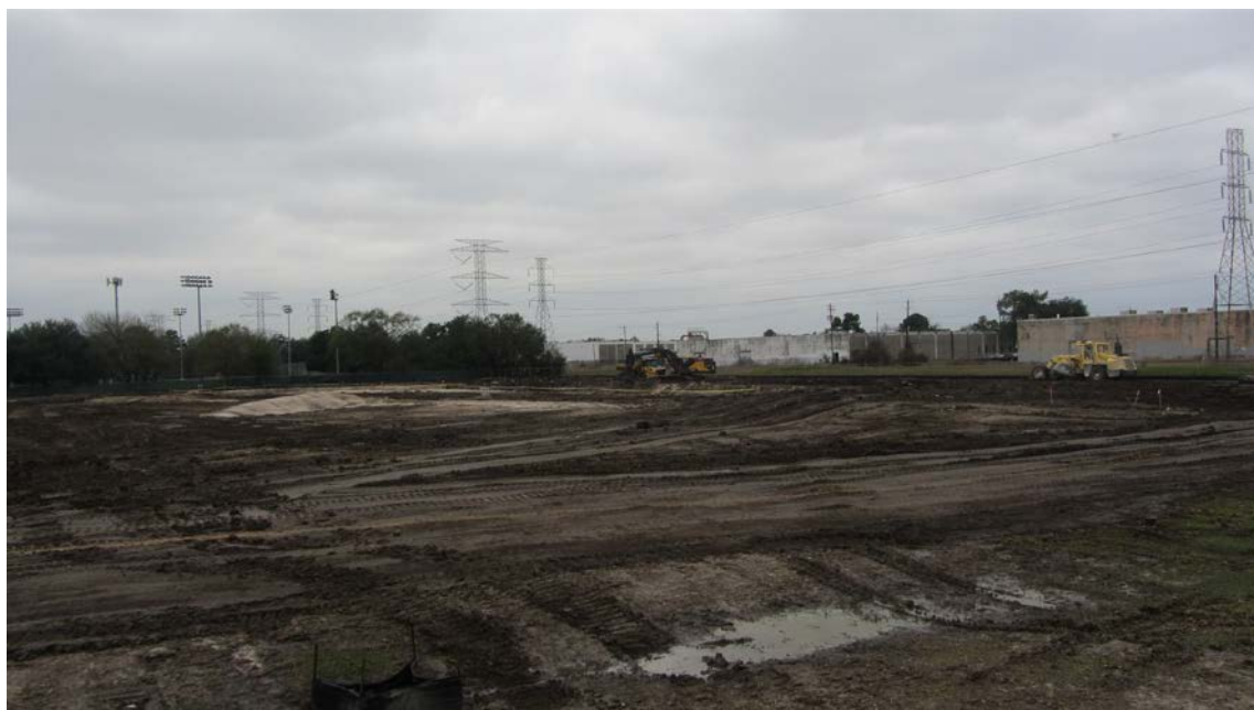
Site Earthwork ongoing.
