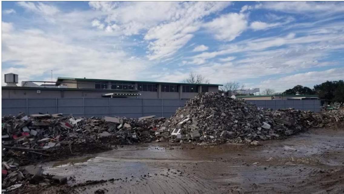
Demolition of Gymnasium complete.
