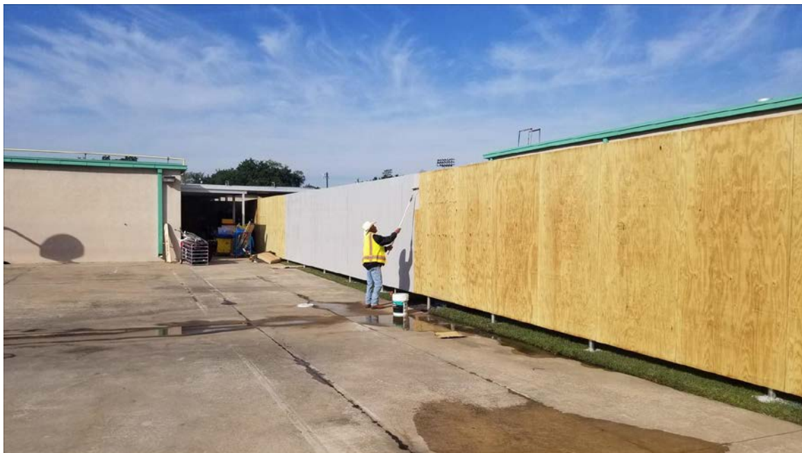
Temporary Construction Fence
