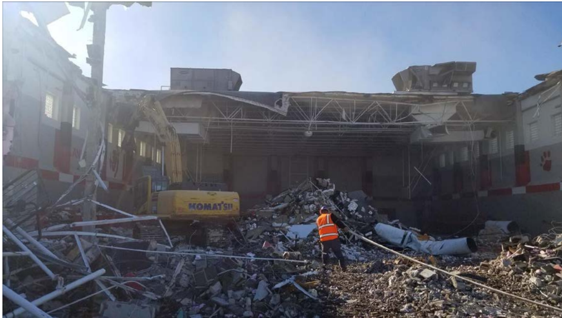
Demolition of Gymnasium
