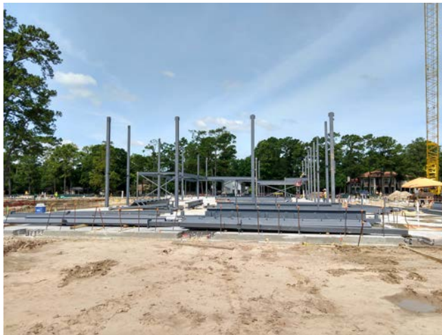
Steel Erecting at Areas 'E' and 'F'
