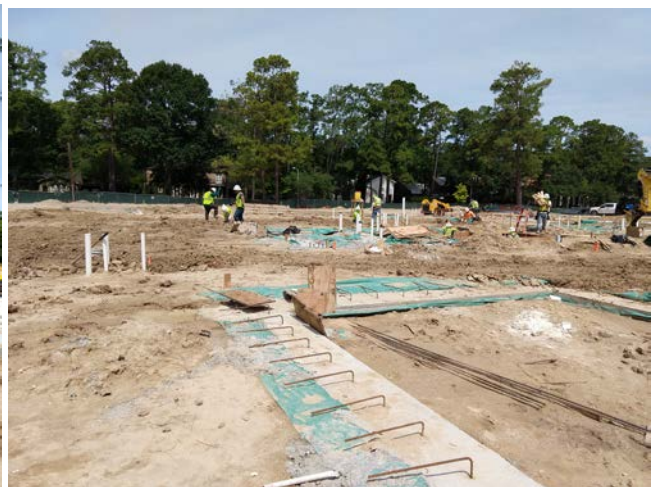
Grade Beam Progress at Area 'D'
