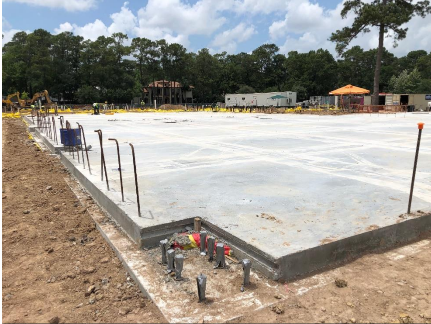
Area E – Slab has been poured.
