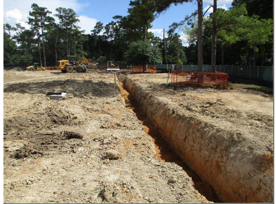
Area F - Domestic / Fire Water Line Installation
