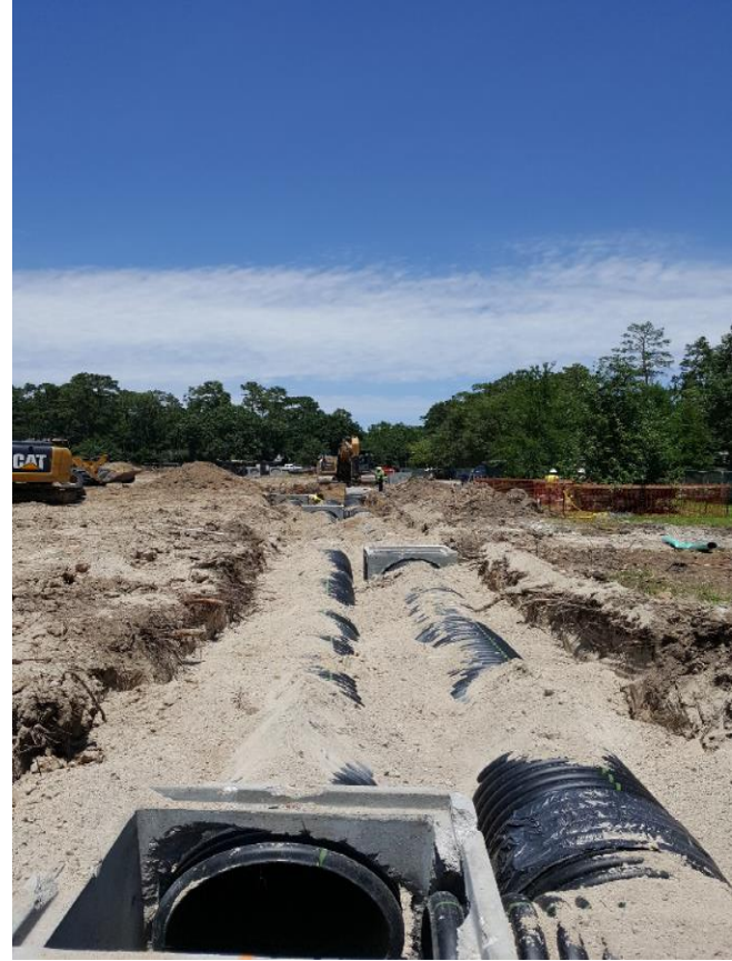
General Site Work: Underground Detention Systems
