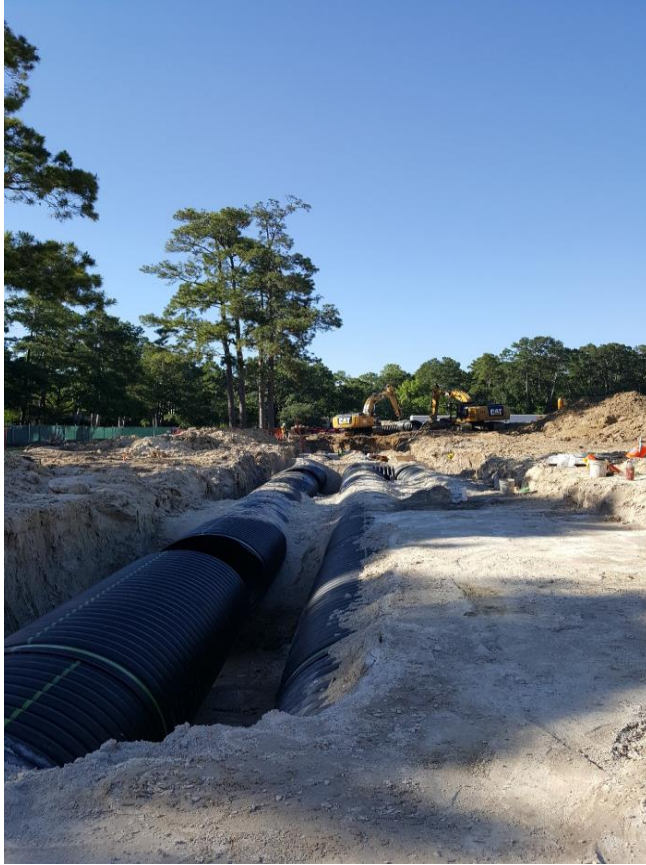
General Site Work: Underground Detention Systems
