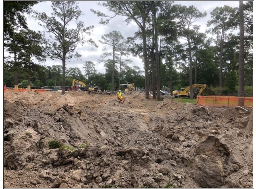
Site & Utility Demolition
