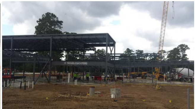
Steel Erecting Progress (Area 'E' & 'F')
