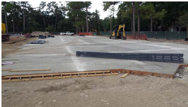
Paving Progress at Bus Loop
