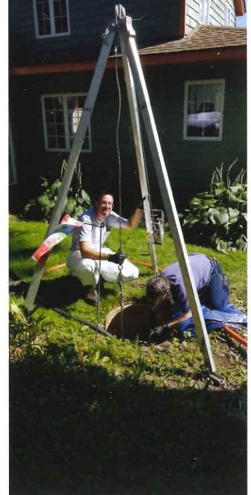
DPW crew members work on servicing/repairing a grinder pump.
