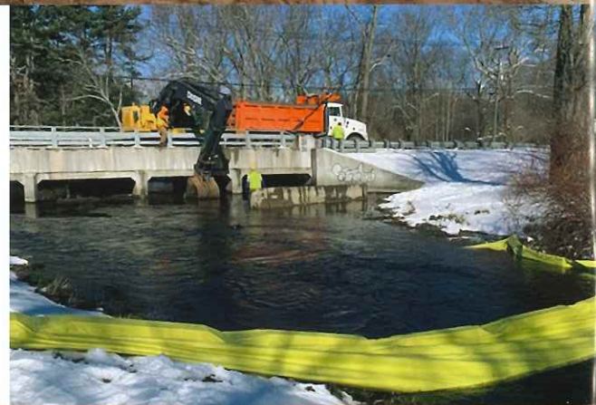
Shown here is a bridge maintenance crew dredging the channel at Windermere Bridge.
