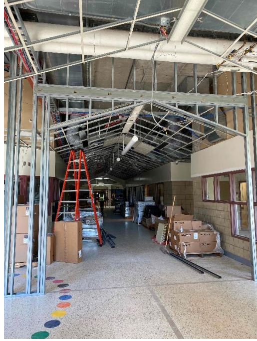
CCES – Framing in progress in new entrance vestibule for area E
