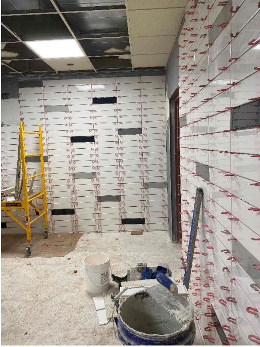
CCES – Tile being installed in bathrooms in area A
