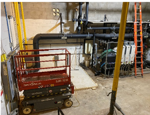
STEM – Boiler Room Mechanical Equipment Concrete Pads
