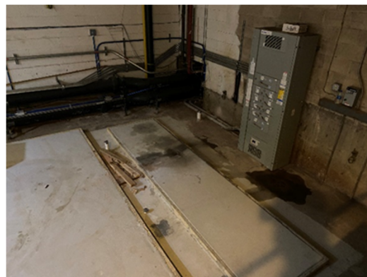
STEM – Boiler Room Mechanical Equipment Concrete Pads
