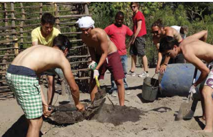
TASIS students mixing termite mud to make the walls of a house for homeless people in Mwandji, Zambia.
