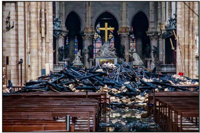
Debris fills the interior of the cathedral after the 12-hour fire.
