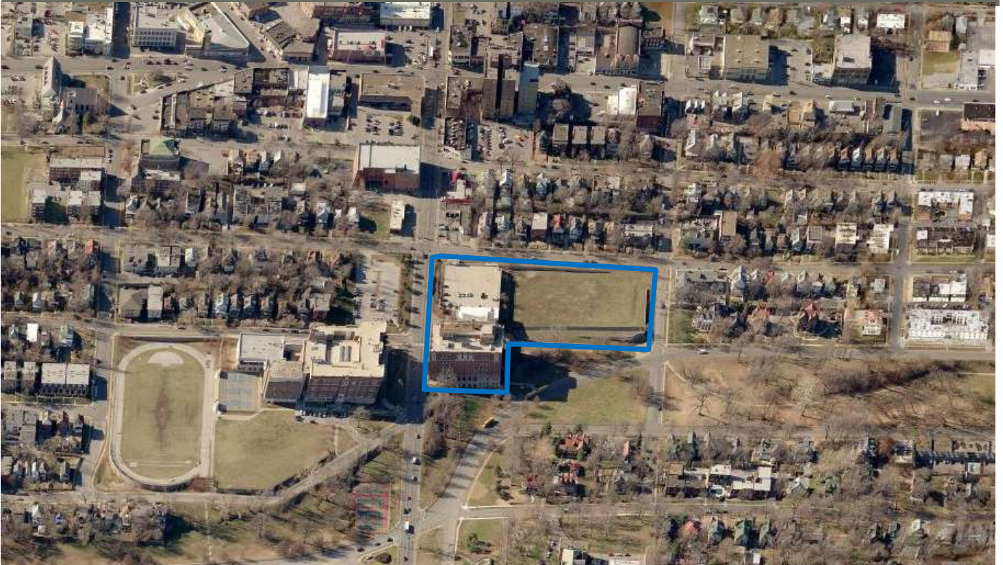
Aerial View: Westport Middle
