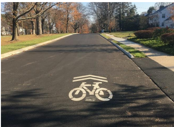
Brookside Boulevard Sharrow Pavement Marking - Looking East
