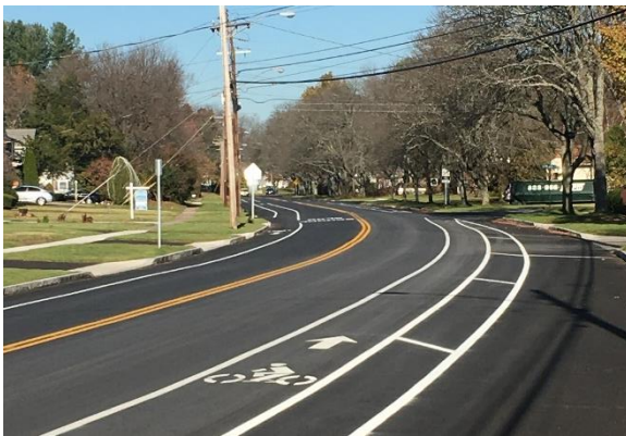
King Philip Drive Buffered Bike Lanes - Looking North just south of Lyman Road
