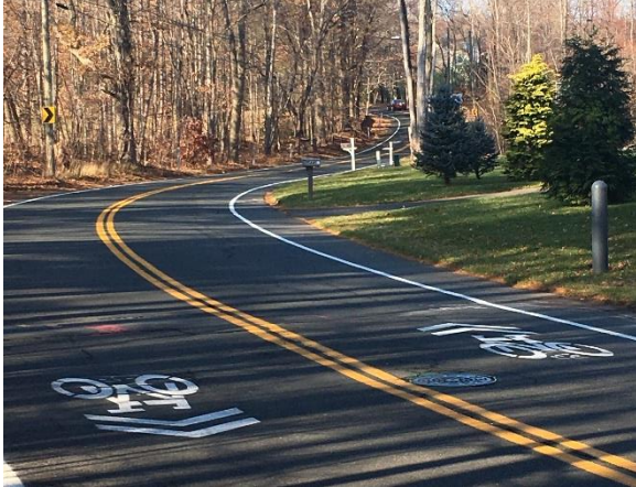
Still Road Sharrow Pavement Markings - Looking West
