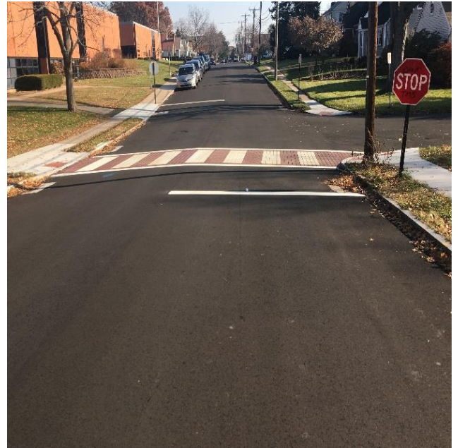
St. James Street Stamped Asphalt Crosswalk Enhancement (In front of the Florence E. Smith Elementary School)
