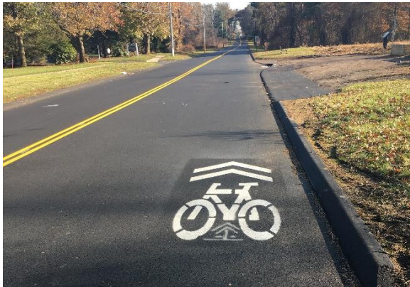
Flagg Road Sharrow Pavement Marking - Looking West
