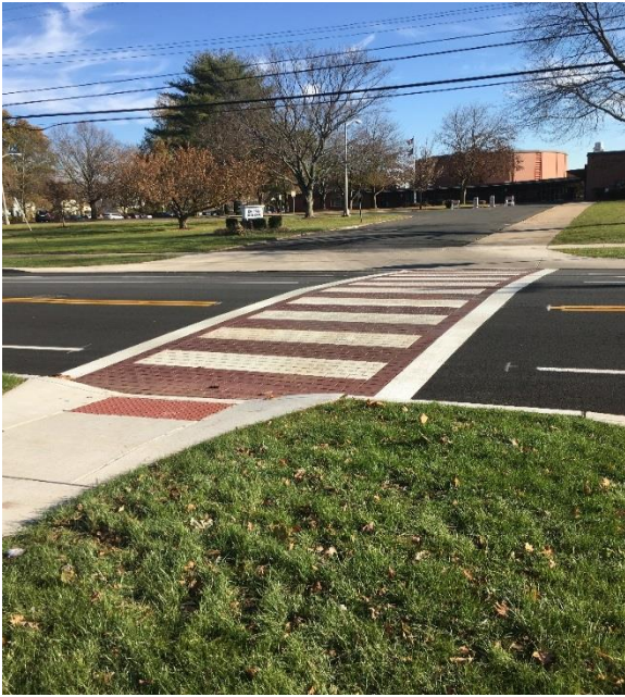
King Philip Drive Stamped Asphalt Crosswalk Enhancement (In front of the King Philip Middle School Entrance)
