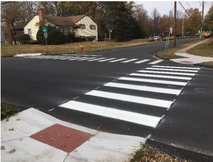
Hilldale Road at Peyote Road Crosswalk Replacement
