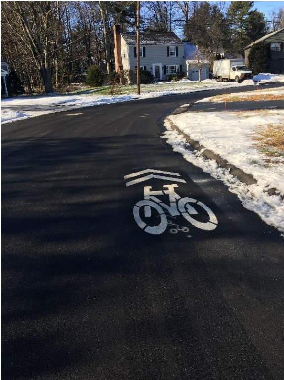
Richmond Road/Day Road – Looking West
