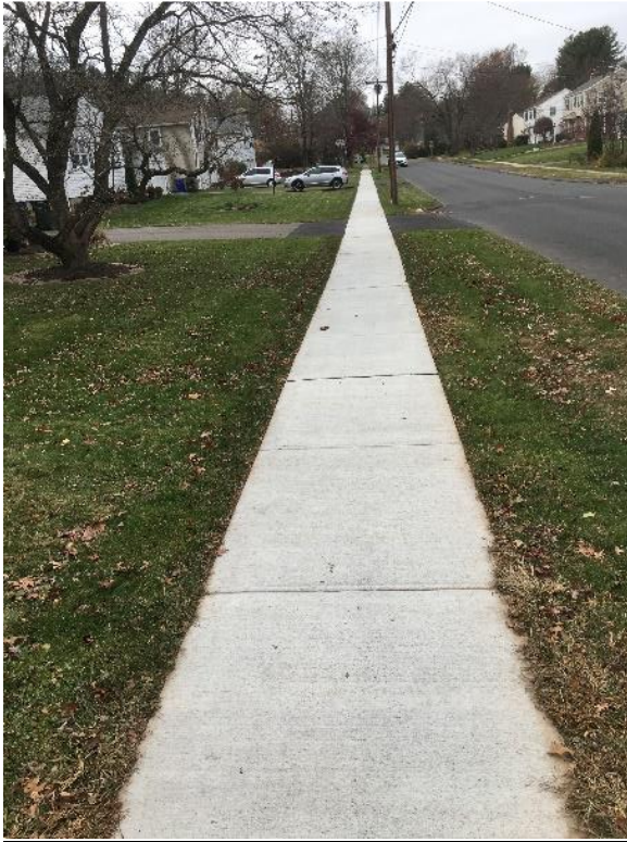
Hilldale Road Long Sidewalk Replacement
