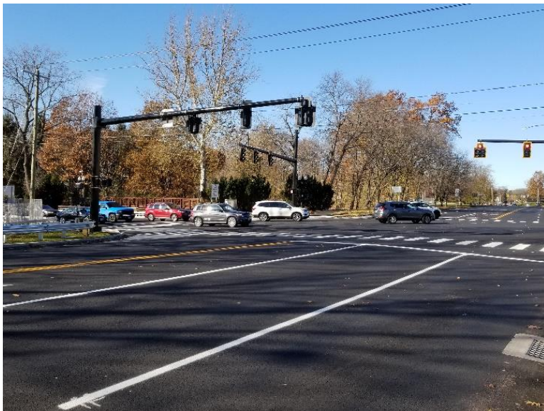
Park Road at Trout Brook Drive - Looking North
