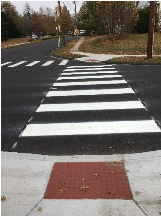
Hilldale Road at Peyote Road Sidewalk Ramp Replacement
